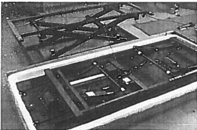
Fig.2.5 Electr. connection of HiLo lifting motor completed.
